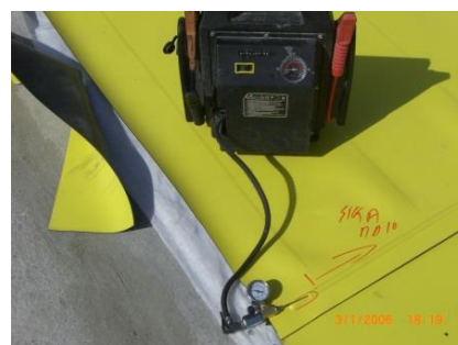
Pressure test of a double seam with an electronic pump
