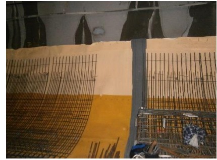
Membrane termination min 200 mm over starter bars
