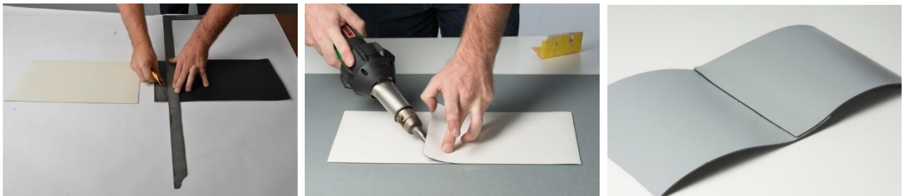
Joining two WP Tapes with overlap welding
