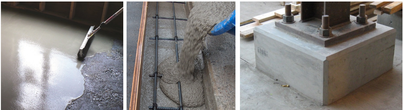
Figure 1: Cementitious components on site
