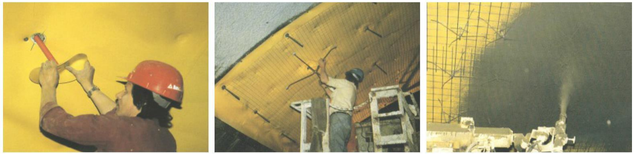
Figure 10: Installation sequence of the Sika Anchor system
