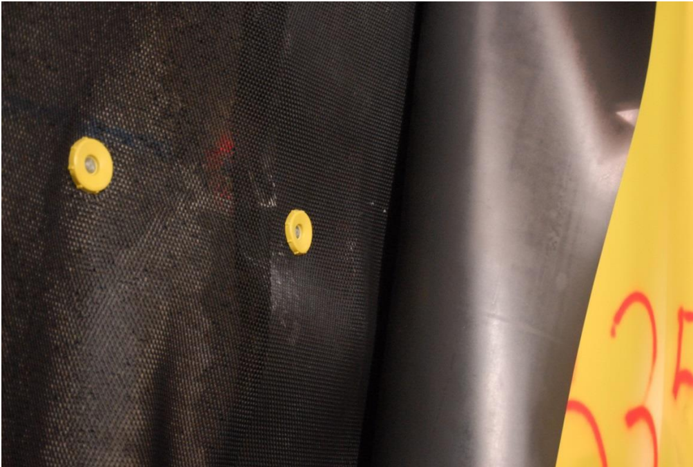
Figure 6: Detail of Sikaplan® W Tundrain (black perforated surface), with Sikaplan® WP Disc 80/10mm yellow (yellow round discs) and membrane layer (black and yellow)
