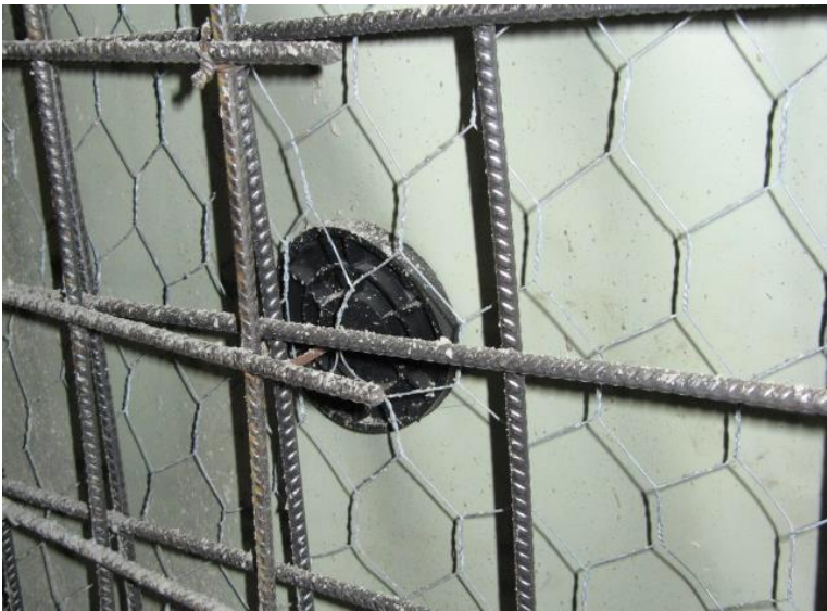
Figure 16: Chicken wire mesh fixed with contra discs
