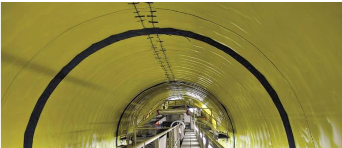
Figure 8: Longitudinal injection hoses on the top section of the sheet membranes
