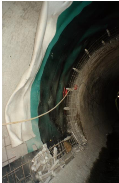
Figure 26: Over-spraying of waterproofing membrane (green), texture achieved by PE-mesh (black), self-supporting steel mesh on top
