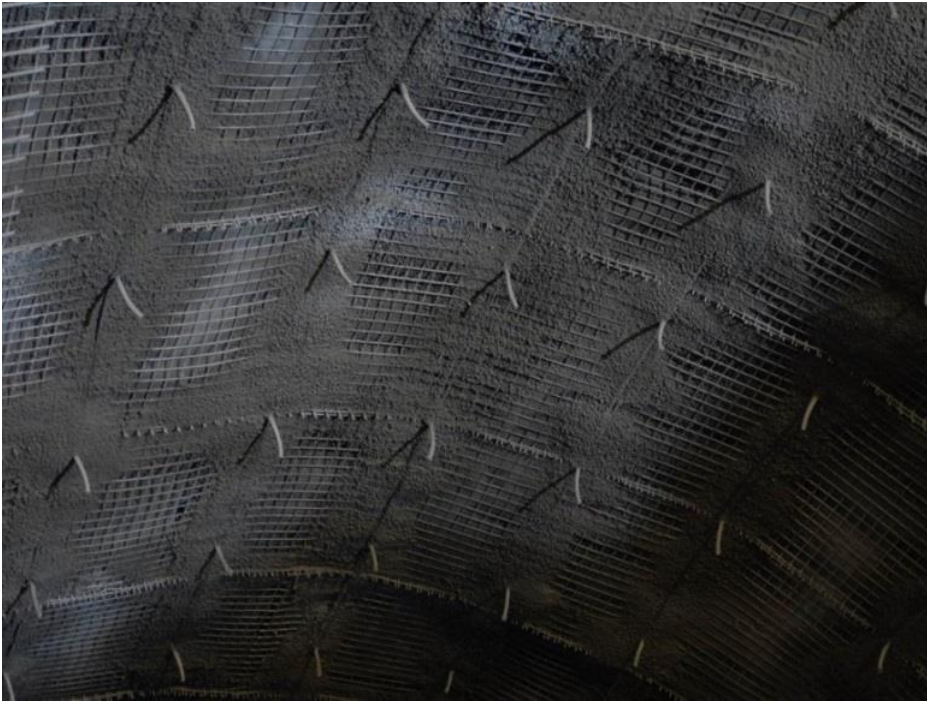
Figure 24: Detail of the steps followed to spray the waterproofing system structure
