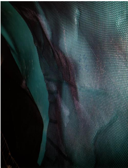
Figure 26: Over-spraying of waterproofing membrane (green), texture achieved by PE-mesh (black), self-supporting steel mesh on top
