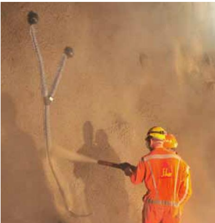
Figure 3: Fixing of Sika FlexoDrain® W with SikaShot®-3
