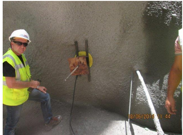
Figure 11: Pull out test STEP tunnel Abu Dhabi
