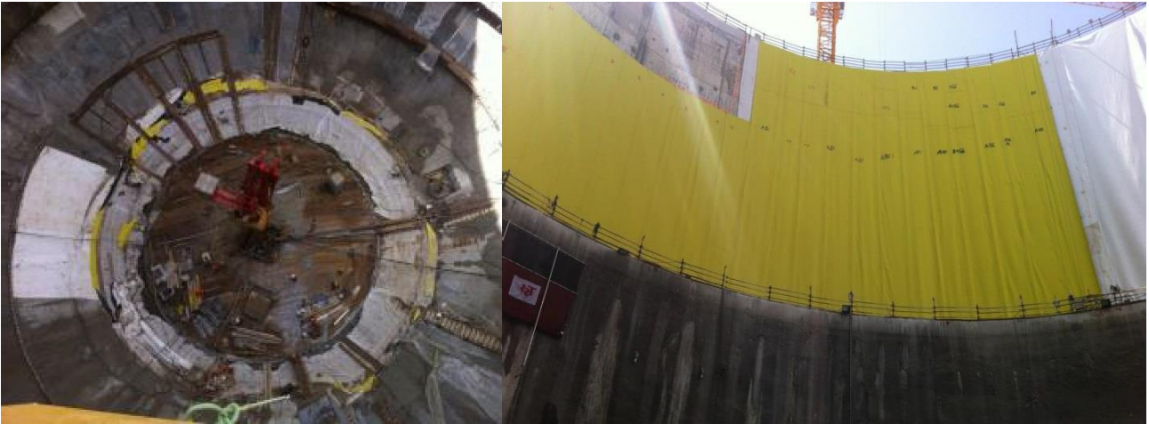
Figure 27: Shafting for the STEP tunnel, Abu Dhabi
