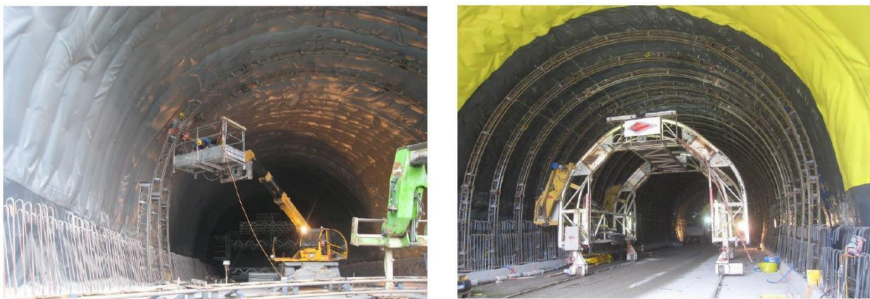
Figure 14: Installation sequence of self-standing / self-supporting reinforcement
